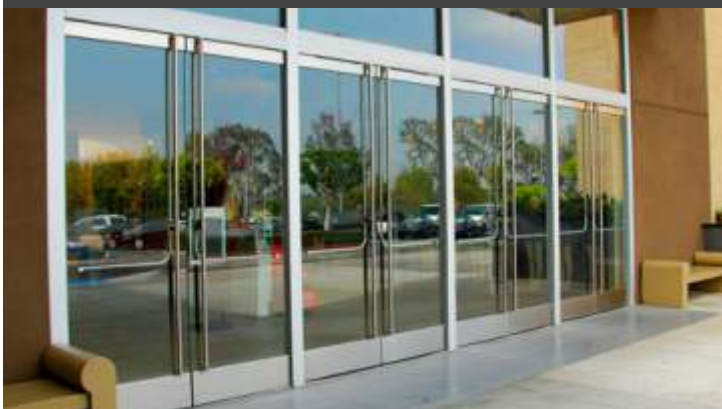
T&A at Entrance area
